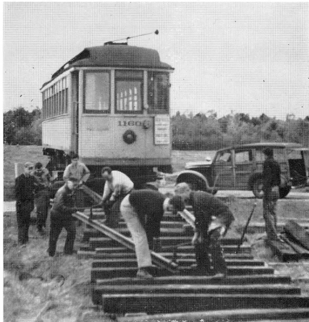
NO. 1160 in the background as Seashore members build ramp for unloading.
