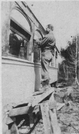
Gene Cote removing paint from 38, preparing car for complete refinishing
