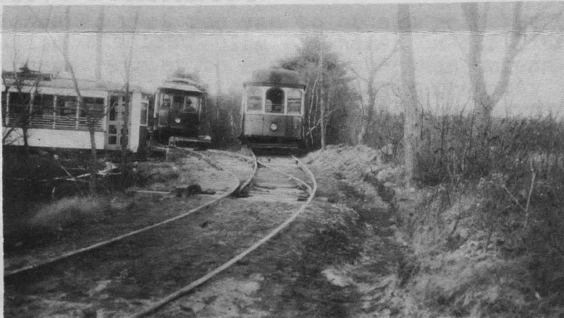
Looking toward the eventual car house lead, from where #60 now stands. Picture by Dan Twomey.
