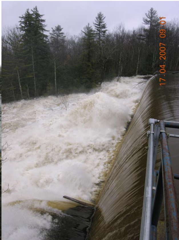
Old Falls Dam before and after the storms.
