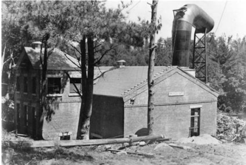
Old Falls Under Construction
